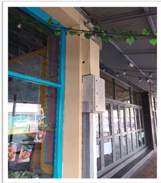
Image 21 - Fuse box cover fixed
