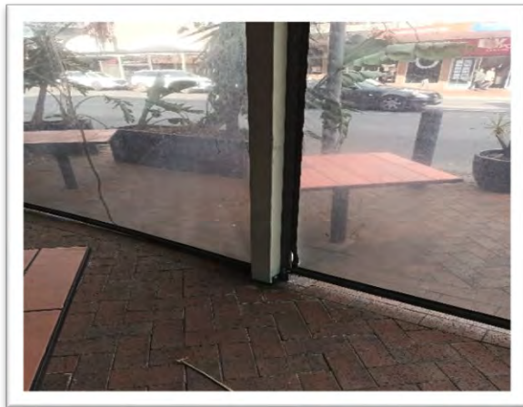
Image 25 - Damaged footing fixed
