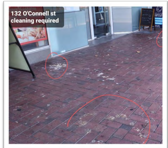
Image 33 - Concentrations of bird droppings under roosting areas
