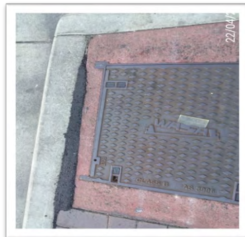
Image 2 - After photo showing cold mix asphalt in place.
