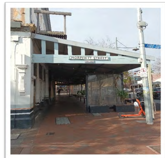
Image 23 - Loose railing fixed.
