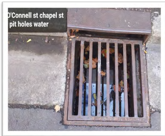
Image 52 - Catch pit holding water.
