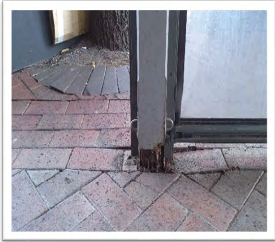
Image 24 - Damaged footing
